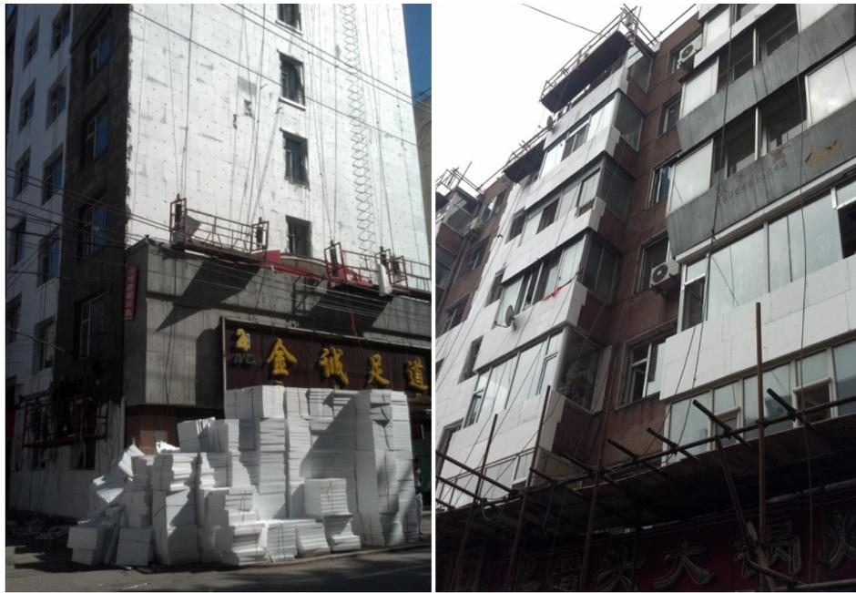
Fig. 1. Buildings undergoing insulation retrofits in Changchun.
